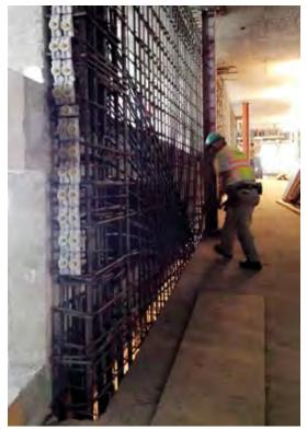
Steel and cables in the post-tensioned beam
