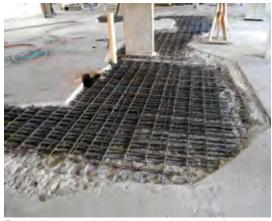
Fourth-level transfer slab crack repair after demolition
