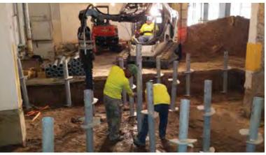
Helical pile installation in the foundation area
