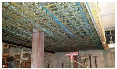
Post-tensioned drop panels with formwork
